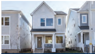
TRI POINTE HOMES Lot 106: 489 Wendover Pkwy
