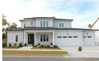
WALKER DESIGNBUILD 65 Edgefield Street - Lot 23
