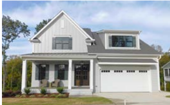
UPRIGHT BUILDERS 63 Cottage Way - Lot 4
